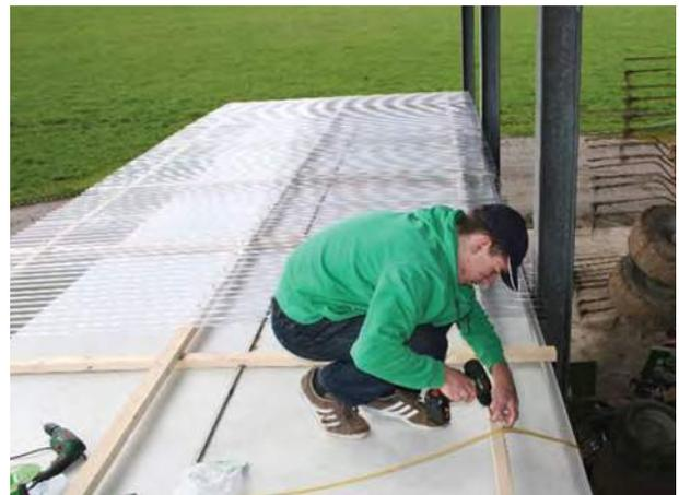
My original idea was using canopies which would have led to adding 3 canopies to the container in total... instead I decided to add a roof construction to the whole container. On top of a simple wooden structure corrugated plastic plates were screwed. The simplest and cheapest solution. At least I thought that at the time. Also more on that later...
